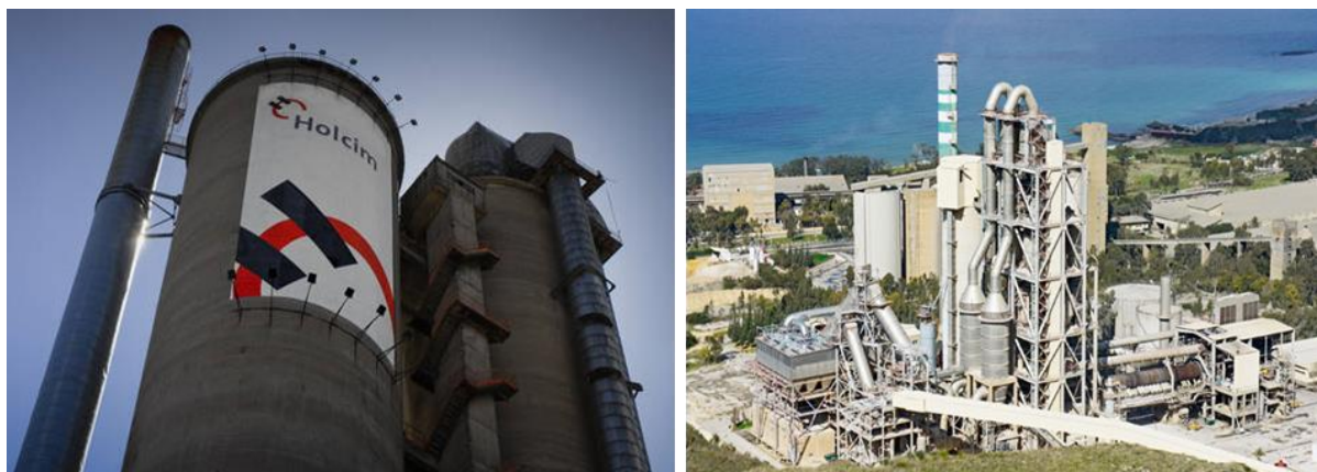
Fig. II-4: Cement plants in Chekka region
