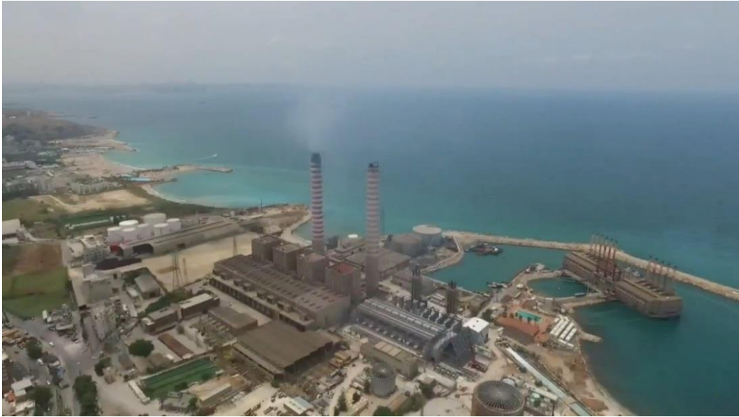
Fig. II-1: The Zouk power plant taken in 2015 by Dark Matters Entertainment
