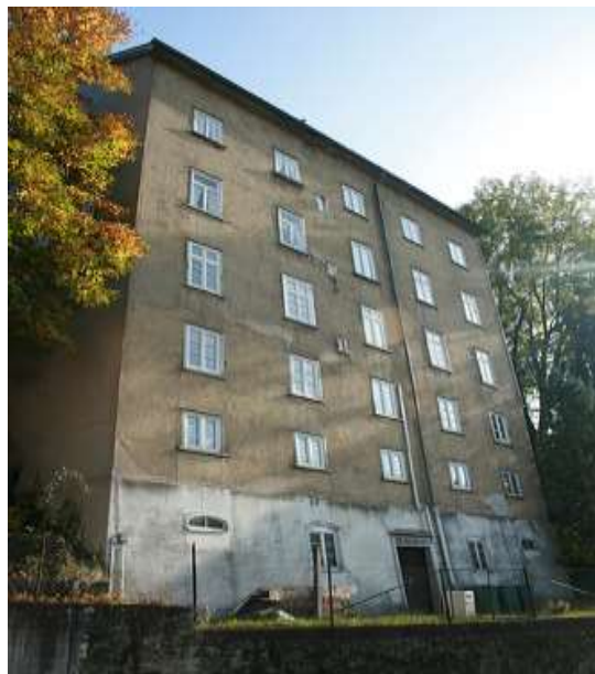
Figure 1.2. Example of modern rammed earth building: the Haus Rath in Weilburg an der Lahn, Germany, built in 1828
