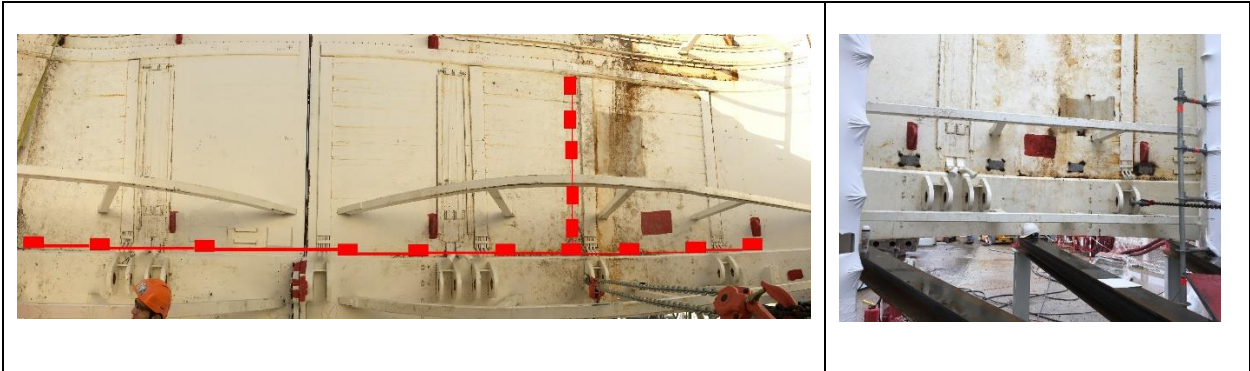
Figure 4-2 Placement of chain nodes (proposed for installation on longitudinal and transversal section)
