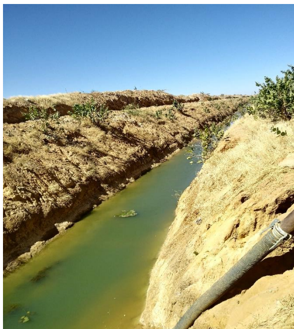
Figure 18 : Canal d'irrigation, Photo KA
