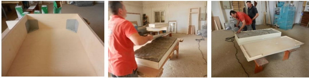
Figure 70. Pictures of the GDC wall prototype made in Herzegovina. Picture left - Wooden box assembly, middle and right – Wooden box with sheep wool. (photo Androšević)
