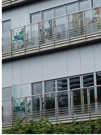
Figure 134 E5 building, detail openings south façade. Source M. Apostolou
