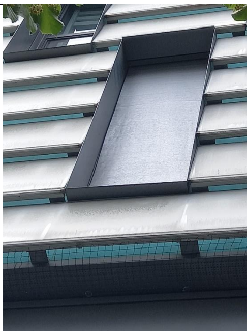
Figure 53 Façade, detail. Building E1. Source M. Apostolou
