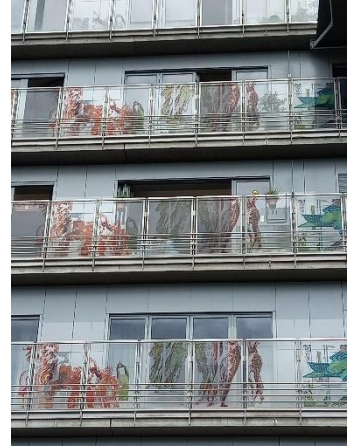
Figure 135 E5 building, detail openings south façade. Source M. Apostolou
