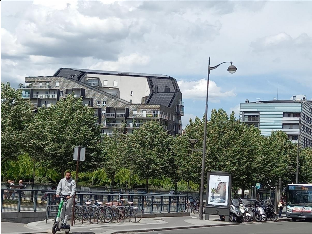
Figure 74 The E2 Building seen from Cardinet street source M. Apostolou
