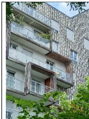
Figure 102 Details, façade. Openings and balconies. Source M. Apostolou
