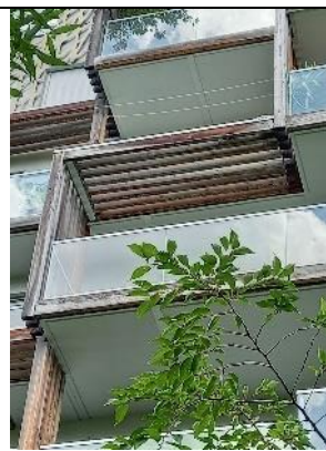
Figure 105 Details, façade. Openings and balconies. Source M. Apostolou
