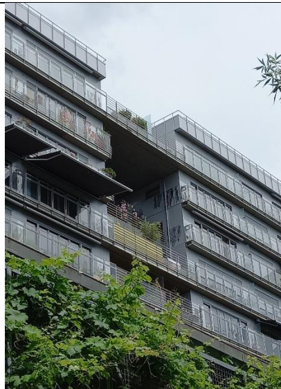
Figure 131 E5 building, fault, south façade. Source M. Apostolou
