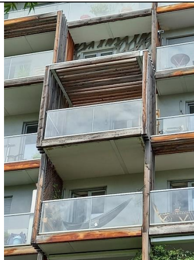
Figure 110 Details, façade. Balconies. Source M. Apostolou
