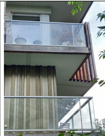
Figure 111 Details, façade. Balconies. Source M. Apostolou
