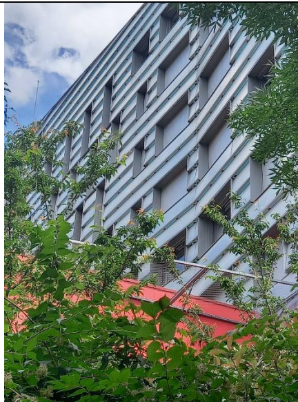
Figure 39 Building E1, View from the park. One can see the creche in red colour. The E1 building is developed mainly along the rue Cardinet, according to a succession of different opaque or glazed elements arranged according to a random rhythm, accentuated by the different colours of the elements characterizing the building's cladding. Source M. Apostolou
