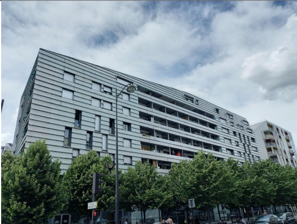
Figure 38 E1 building, south façade, Cardinet street, Paris. Source M. Apostolou
