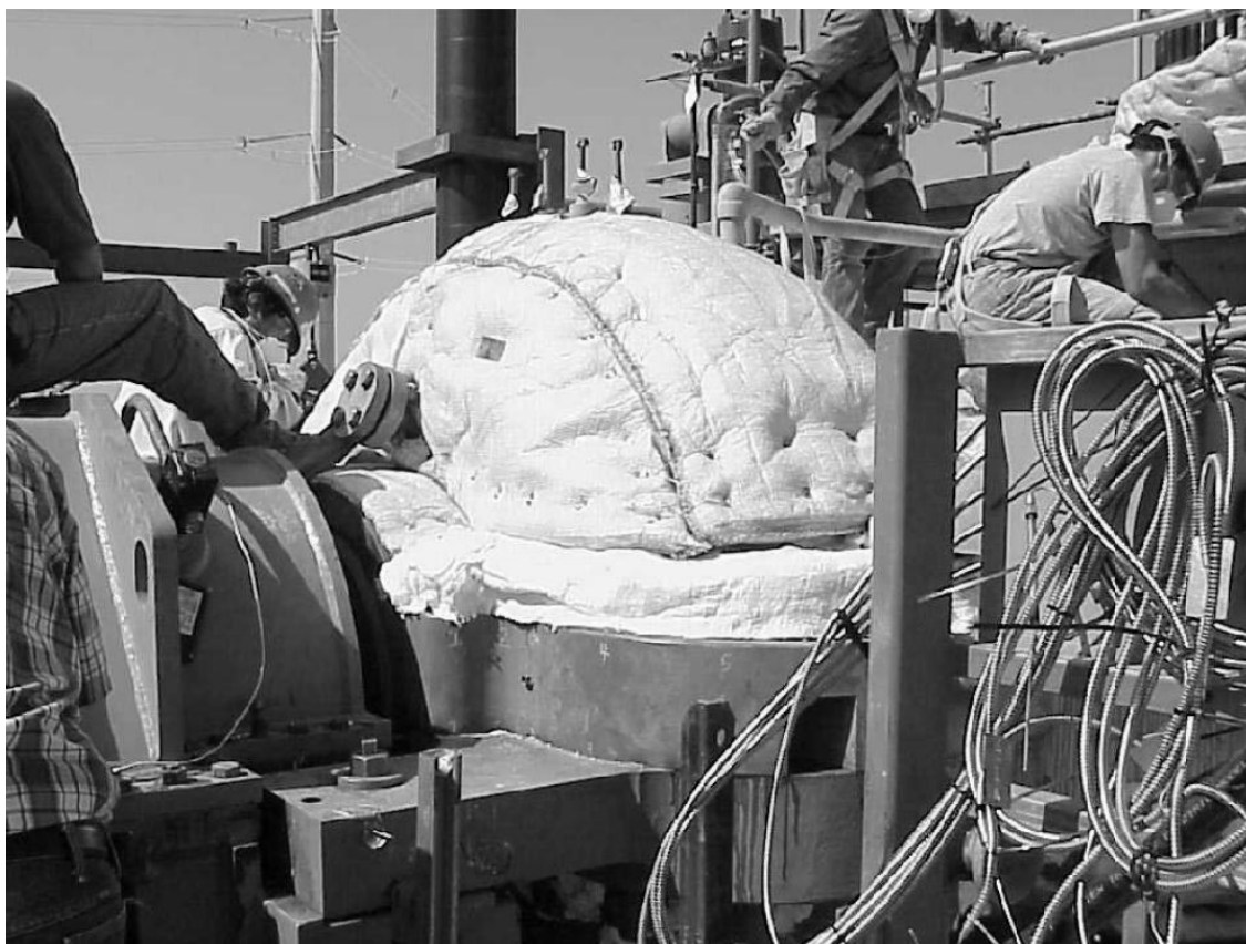
Photo 7 - Top front view of the turbine with inner layer blankets installed.
