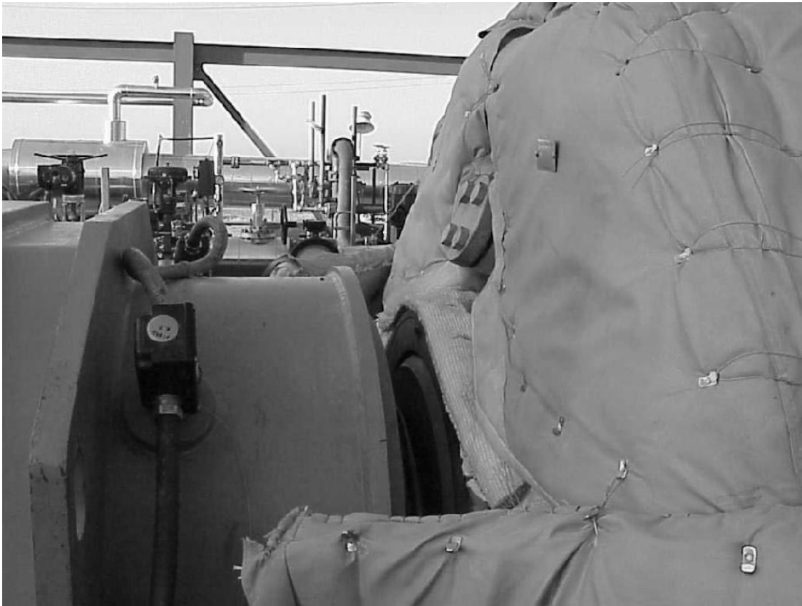
Photo 12 - View of the front bearing housing with inner layer blankets installed.
