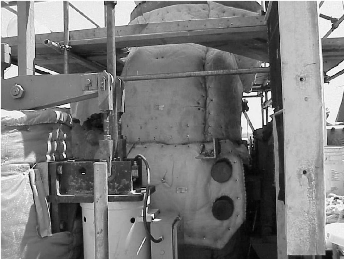
Photo 8 - View of the back side turbine with inner layer blankets installed.
