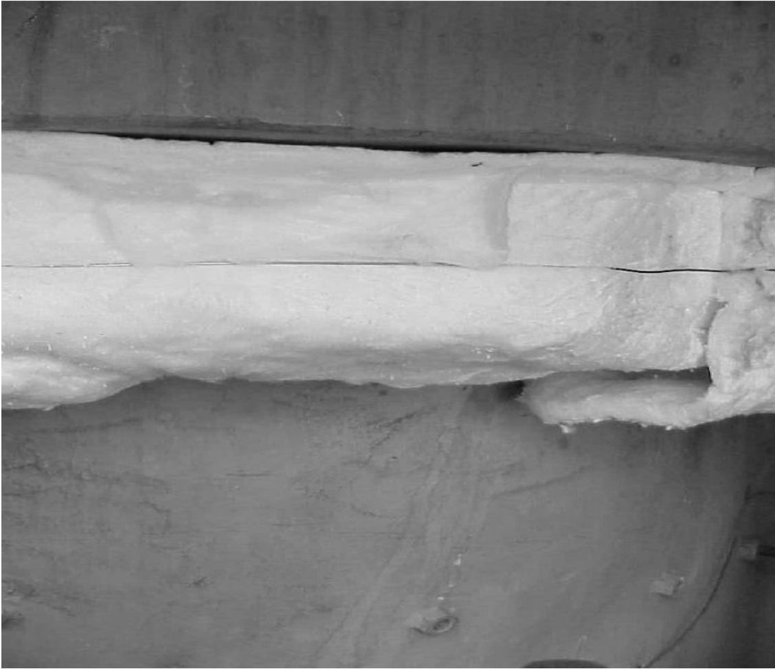
Photo 4 - Horizontal joints covered with required loose mat insulation (1/2 inch thickness).
